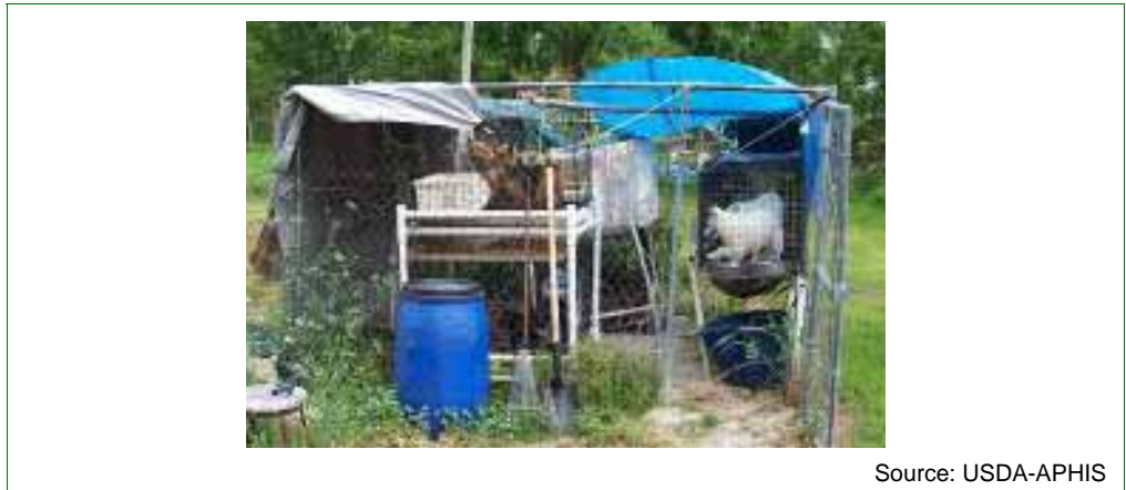
Figure 8-16 Shelter Not Structurally Sound
