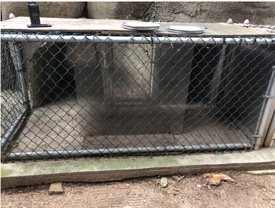
Squeeze portion of the tunnel with the plexi in the middle.
